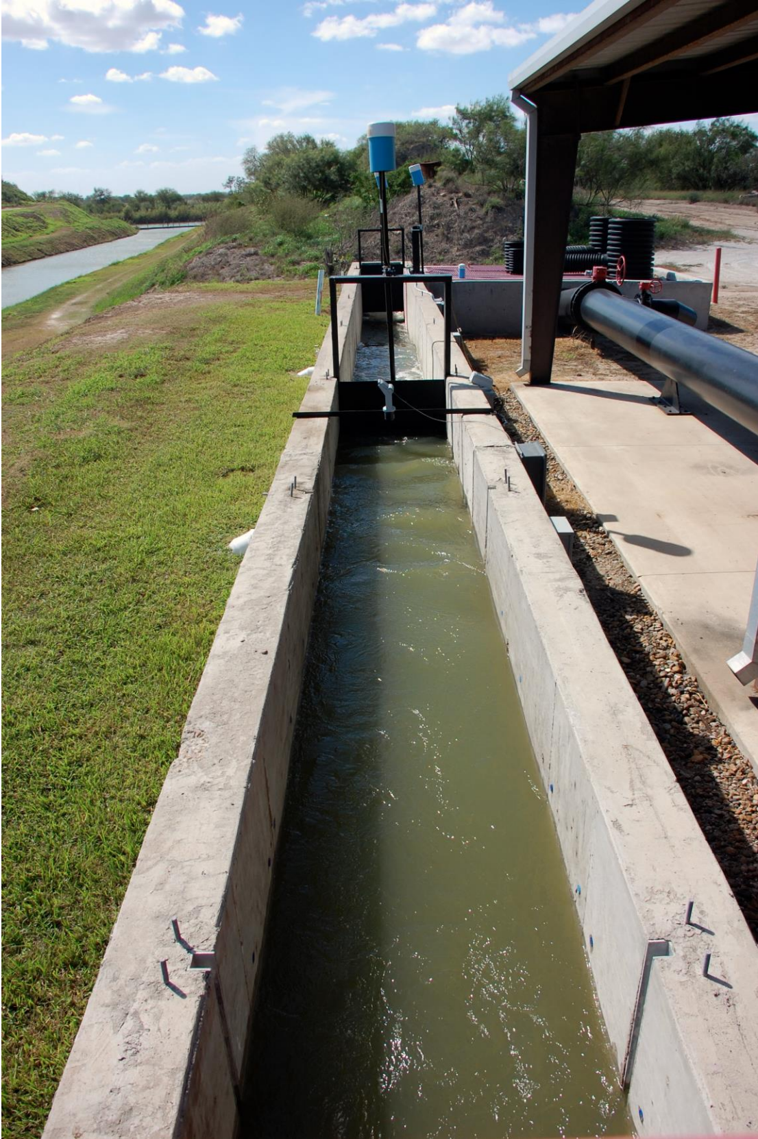
Flume with water showing auto-gate.
