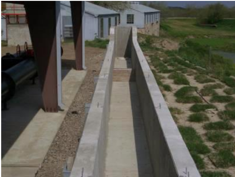
Flume inlet with sharp crested weir.
