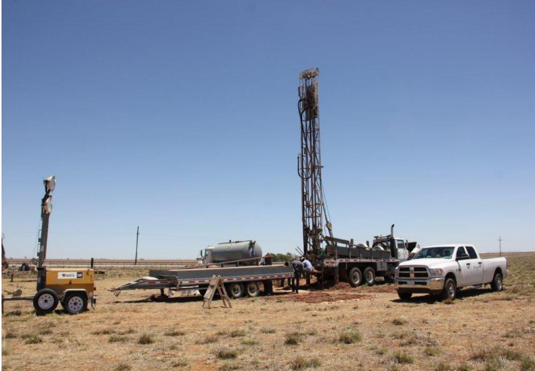
**Figure A-2. The Dockum exploratory test boring drilling site.**
