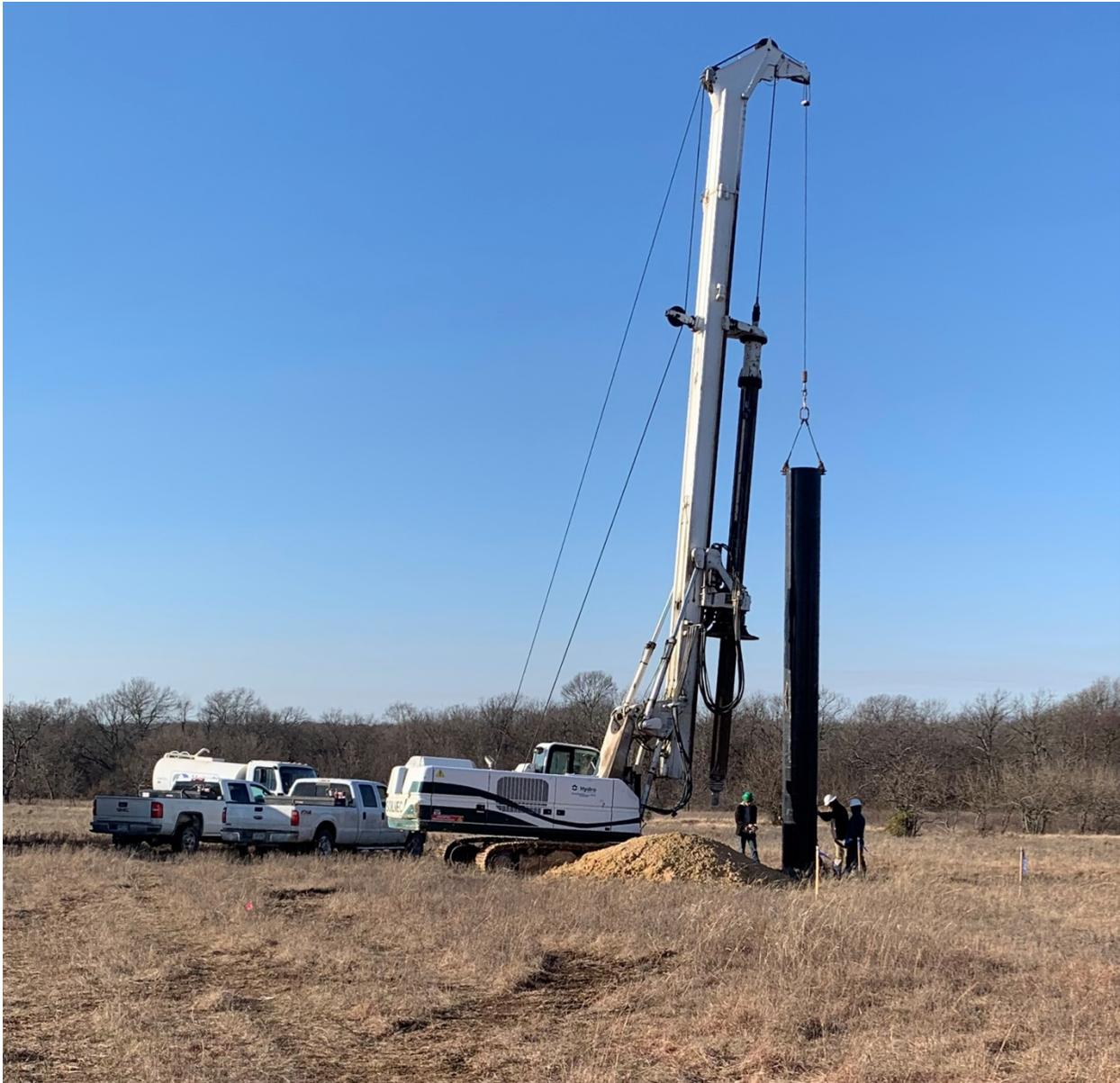
**Figure 3-13. Installing conductor casing.**
