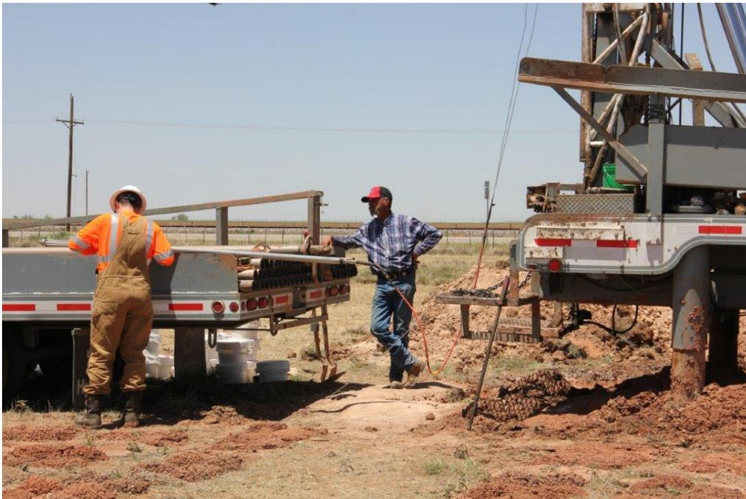
Figure A-5. Preparing a logging tool for use in the exploratory test boring.
