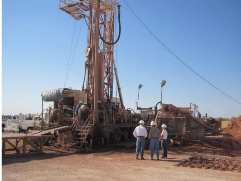
Figure 4. WTWWS drill rig and crew during drilling event
