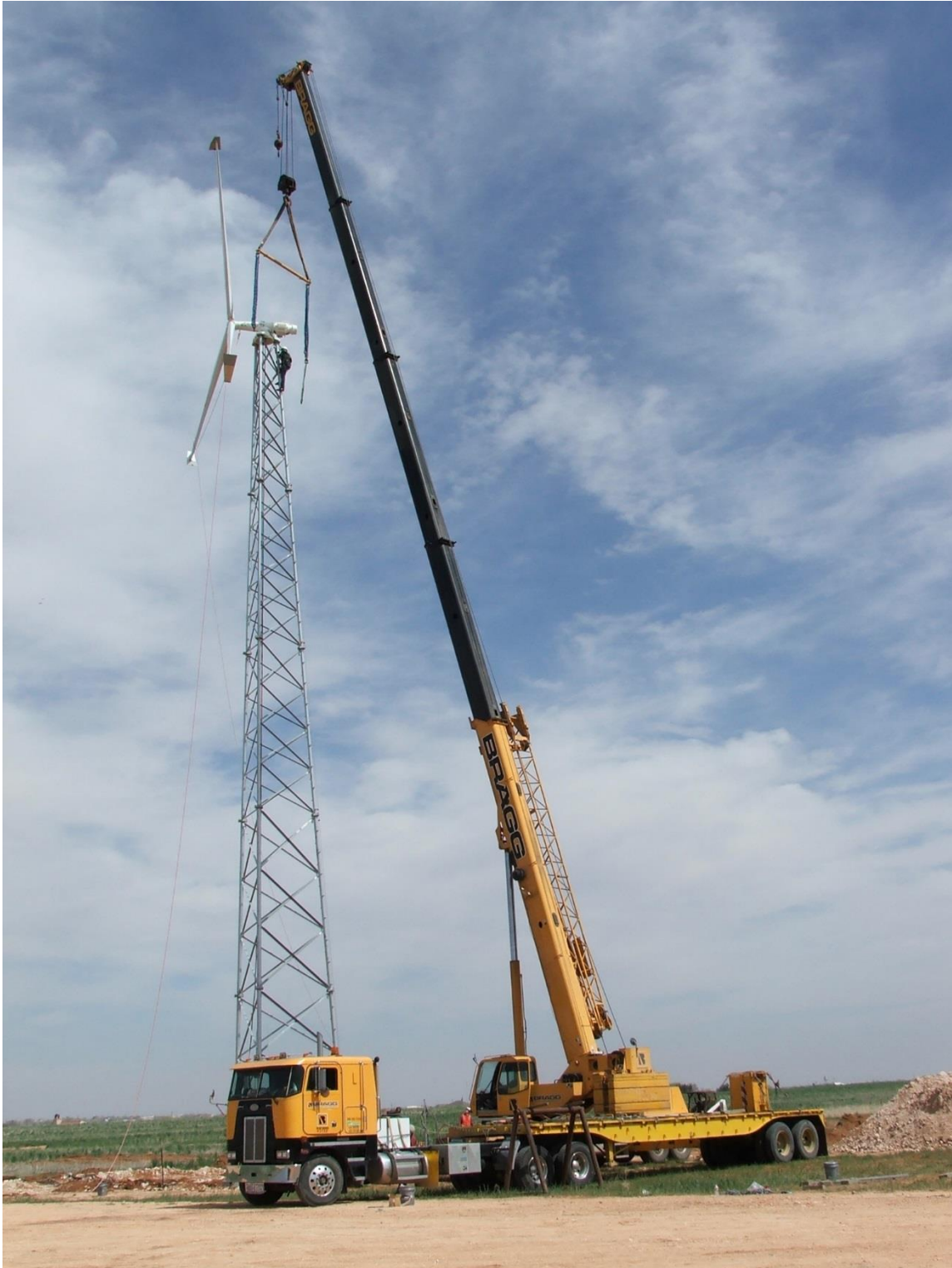
Figure 11. Assembly of the 50-kW wind turbine
