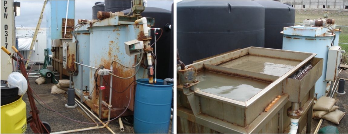
Figure II-10: Conventional pretreatment system (left), and clarifier with settling plates (right).
