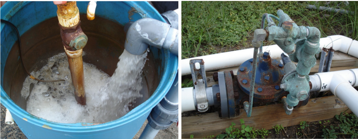
Figure II-8: Raw water coming in from Gulf of Mexico (left), pressure relief valve (right).
