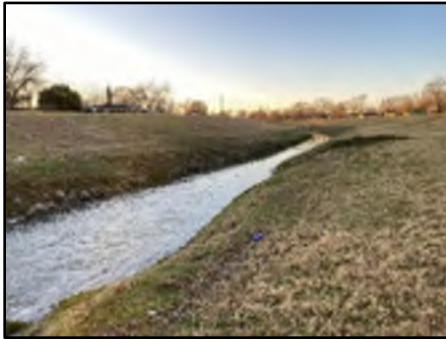
Figure 2-1: Halls Bayou just downstream of Hopper Road
