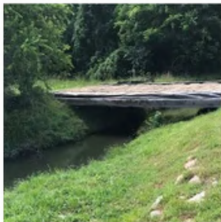
Figure 2-2: Temporary Pipeline Easement Wood Bridge
